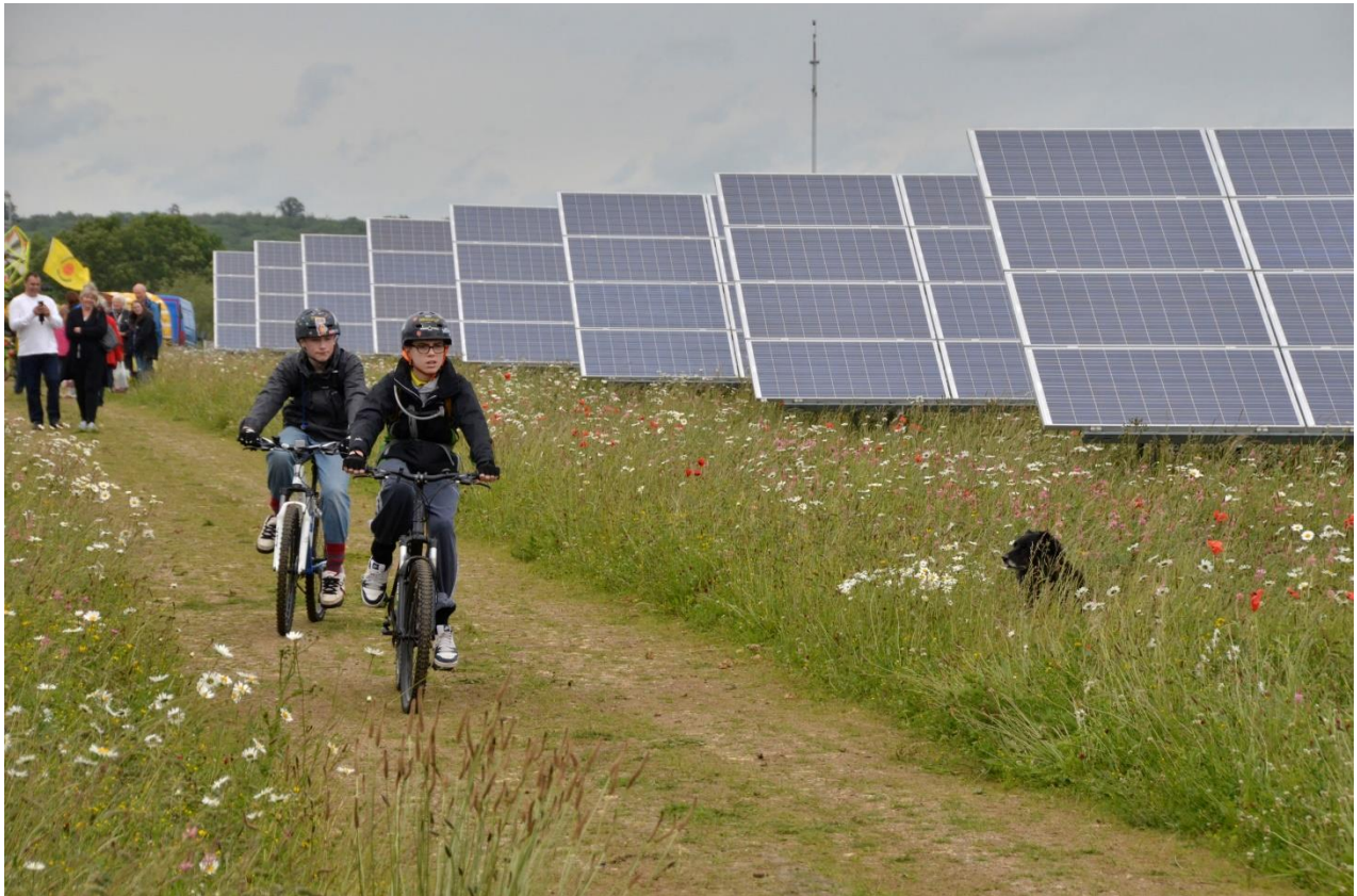
Westmill Solar Park in Oxfordshire: this 5 MW FiTs-supported project was for several years the world's largest community-owned solar power station
